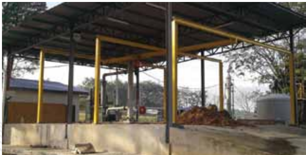
Fig.2 Pool type (scaled-up) self-sustained carbonization reactor
