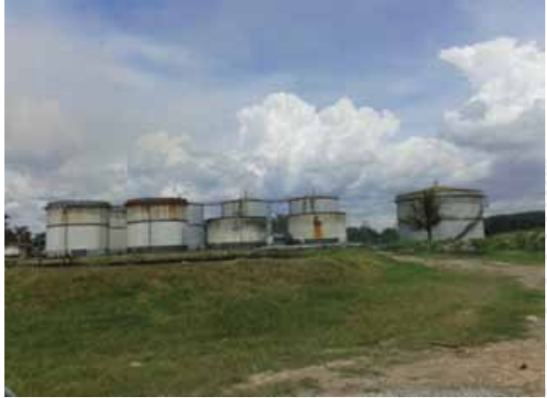
Reactor tank for palm oil mill effluent treatment
