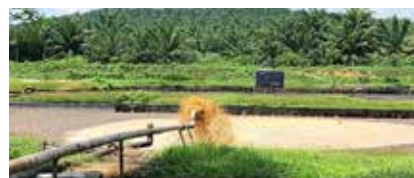
Figure 1: Palm oil mill effluent mixing pond
